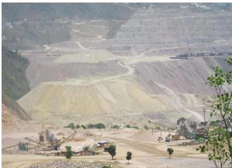
Fig. 35. A view of Koldam (800 MW) hydropower project under construction in the Sutlej basin depicting few of the environmental impacts of hydropower development.
